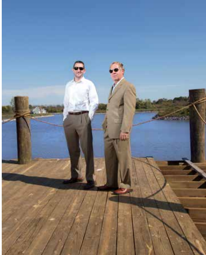
Marty Finta V (left) and Marty Finta IV stand on a Snug Harbor wharf under construction.
